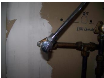
“Schell” shut off valve faucet underneath the bathroom sink cupboard
