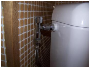
“Schell” shut off valve faucet of the flush tank.
